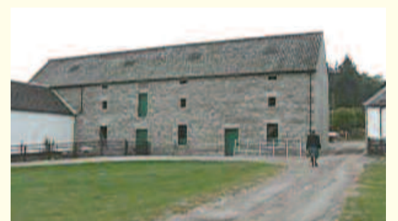
Tulloch Farm: Barn on North side of the Farm Square
