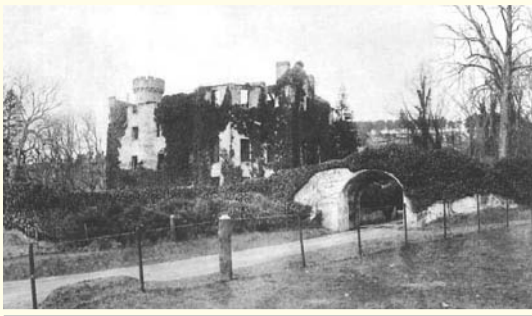
View from the South East pre 1891 Restoration
