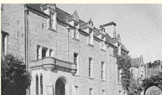
East Wing after 1920 Restoration
