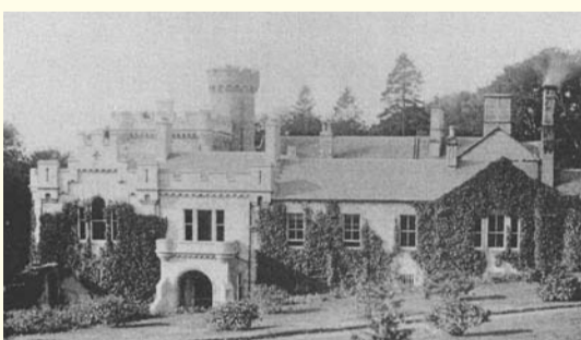
East Wing after 1891 Restoration
