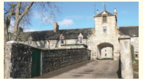
Tulloch Farm: Archway Entrance to Farm Square from the South
